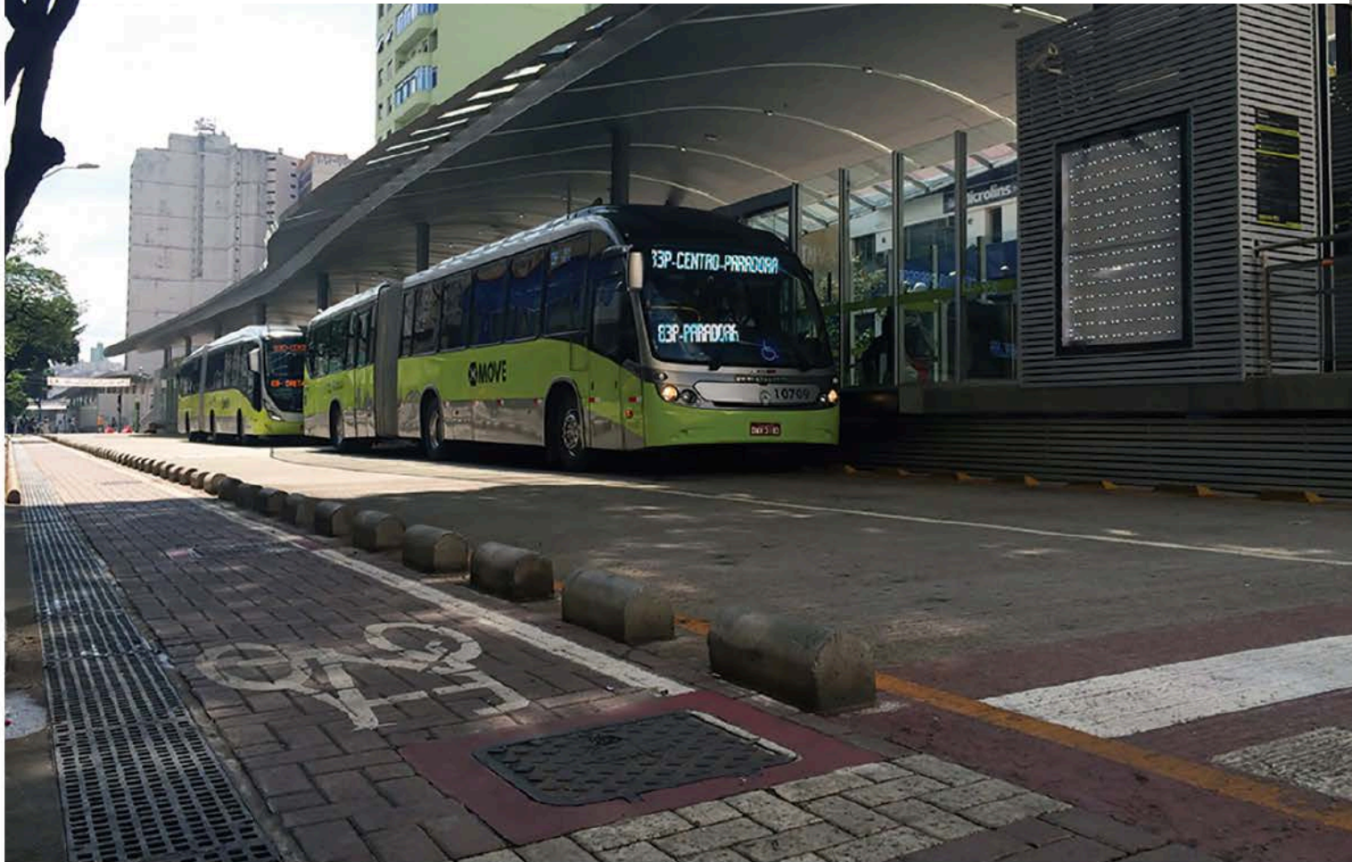
Figure 9.7 Modern bus rapid transit systems can offer high-capacity mobility for medium-density routes at much lower investment than underground metros.
